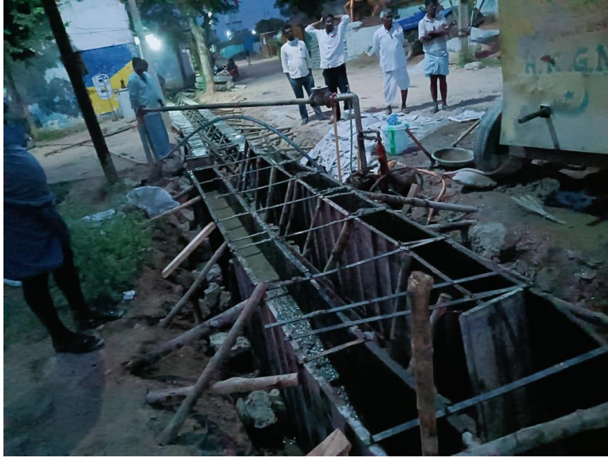
Figure 6. 4 Placing of concrete while construction of open drainage channel at Bollaram village.
