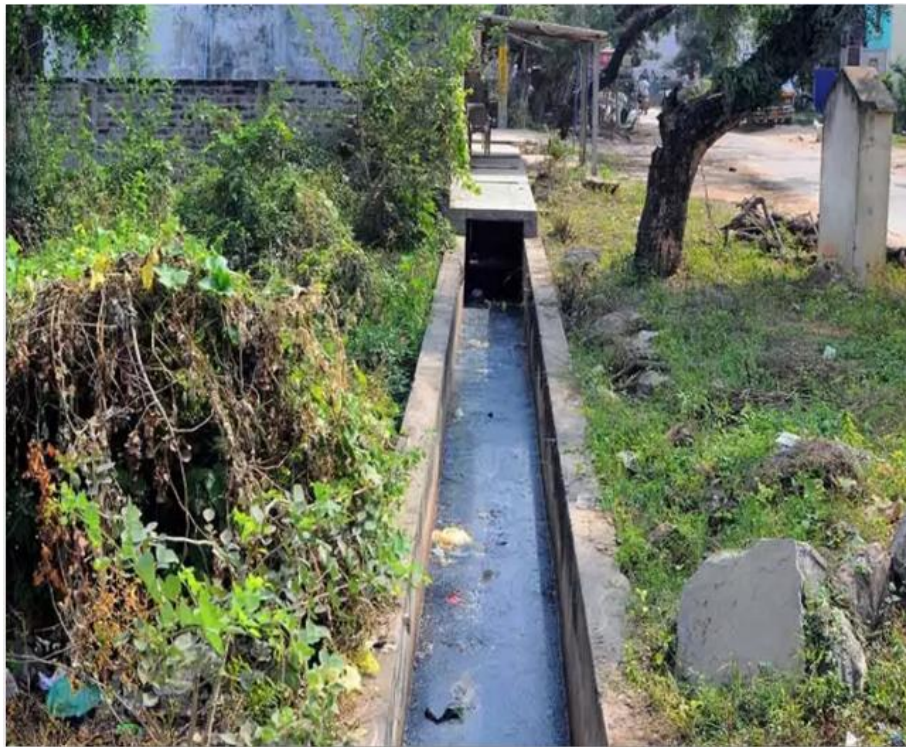
Figure 1. 2 Photo view of blocked drainage channel at Vijayawada
