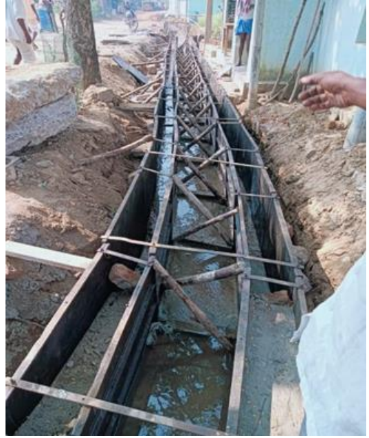
Figure 6. 2 Preparation of formwork to construction open drainage channel by TS Panchayat Raj Dept. at Bollaram village.
