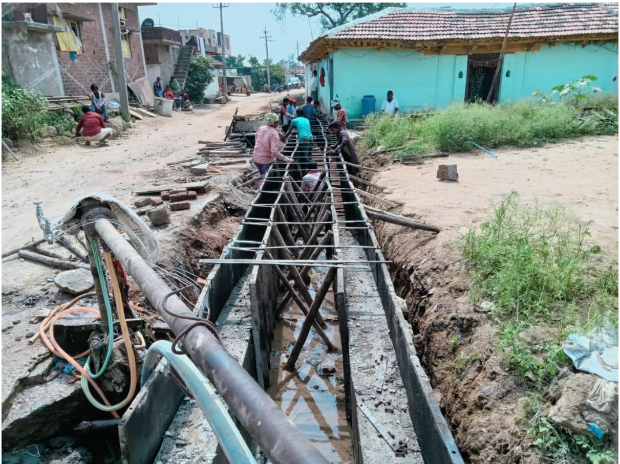
Figure 6. 5 Photo view of under construction open drainage channel.
