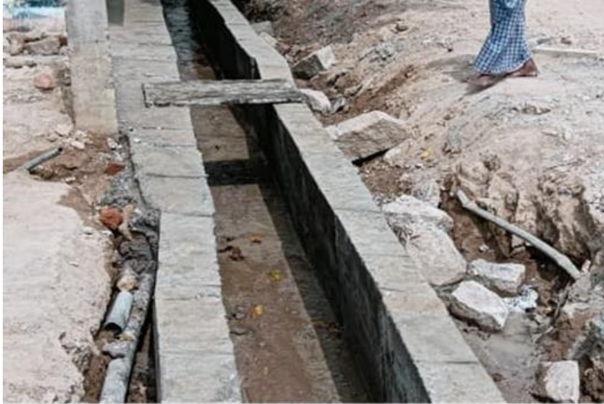
Figure 1. 5 Sedimentation in storm drains during dry weather conditions
