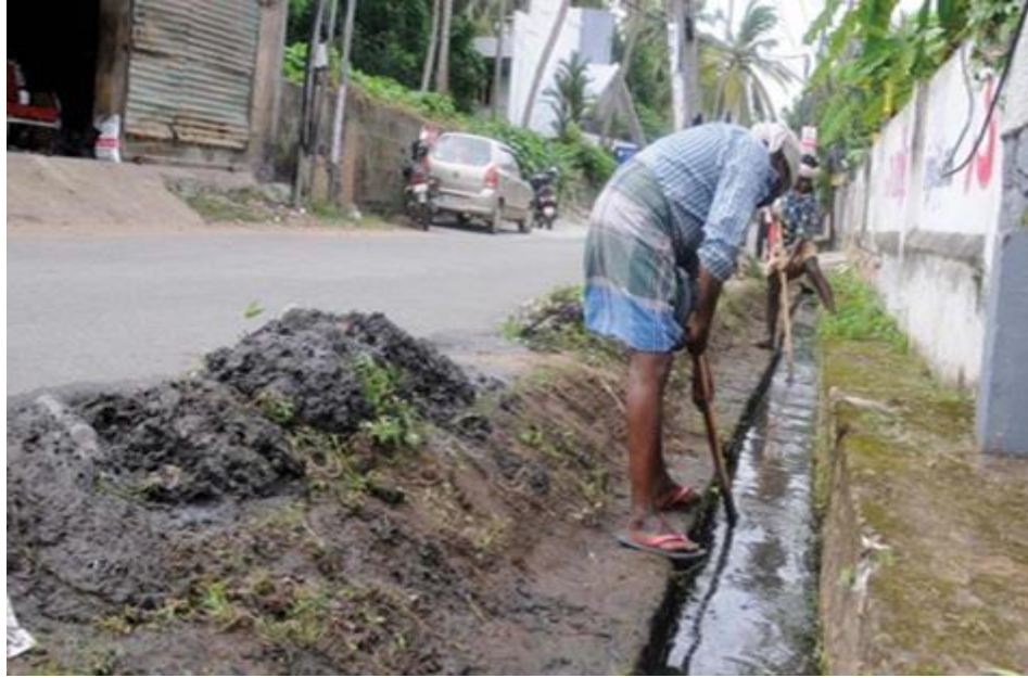
Figure 1. 3 Photo view of desilting of drainage channel at Thiruvananthapuram (India)
