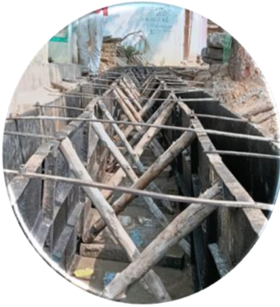
Figure 6. 2 Preparation of formwork to construction open drainage channel by TS Panchayat Raj Dept. at Bollaram village.
