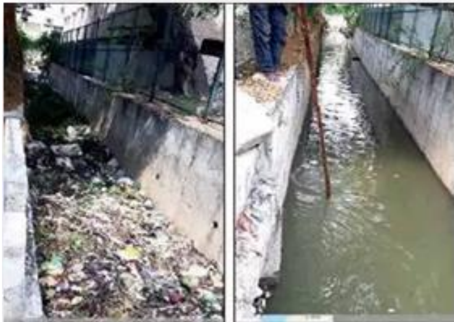
Figure 1. 4 Photo view of drainage flow in blocked channel and cleaned channel at Bengaluru (India)
