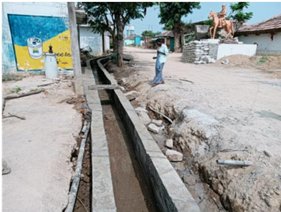
Figure 6. 3 Conventional drainage channel construction by TS Panchayat Raj Dept. at Bollaram village.
