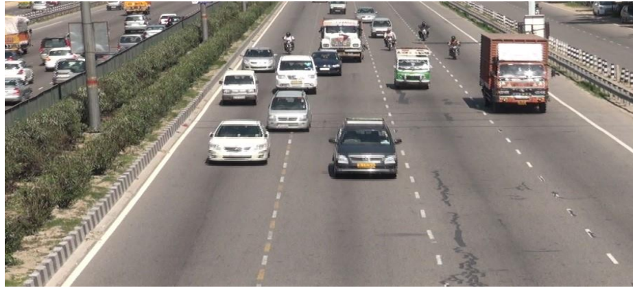
Figure 4.3 Section of eight-lane divided highway with paved shoulder (section-VIII)
