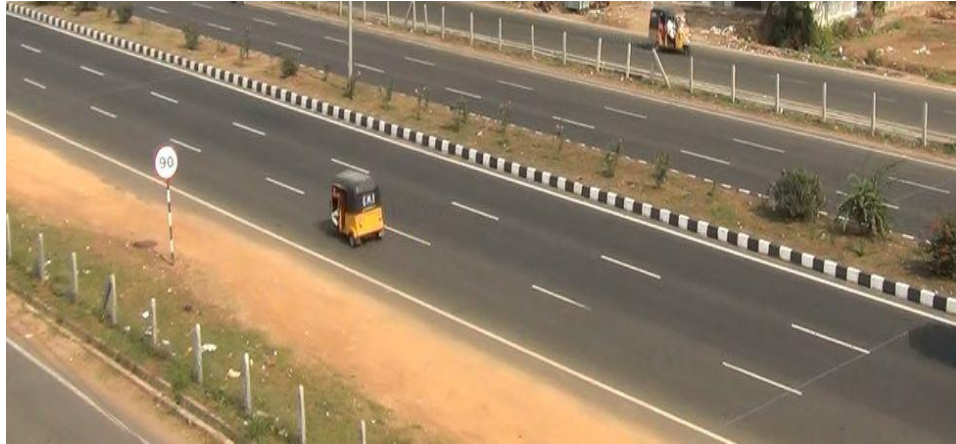
Figure 4.2 Section of six-lane divided highway with paved shoulder (section-VII)
