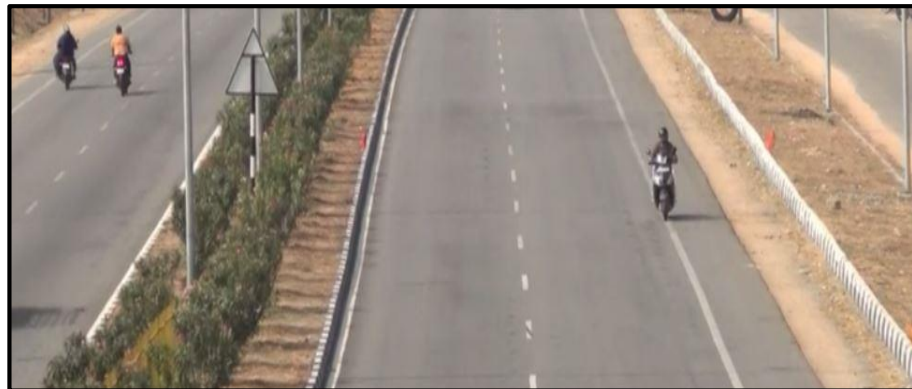
Figure 4.1 Section of four-lane divided highway with paved shoulders (Section-II)
