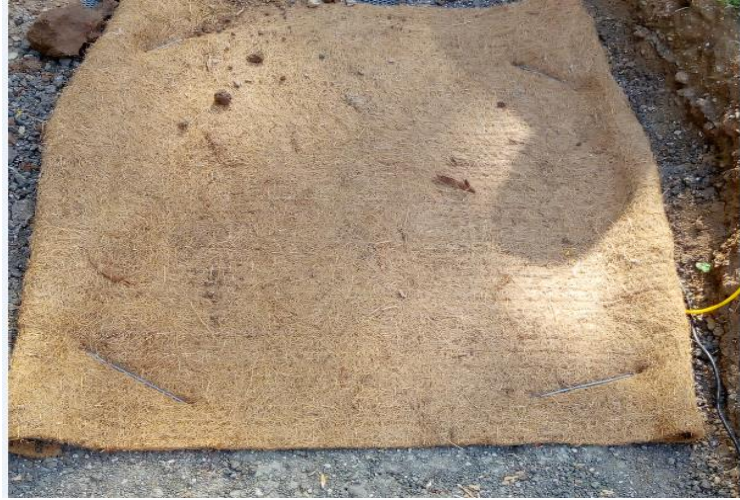
Figure 3.17 Anchoring of coir geotextile mats over the subgrade
