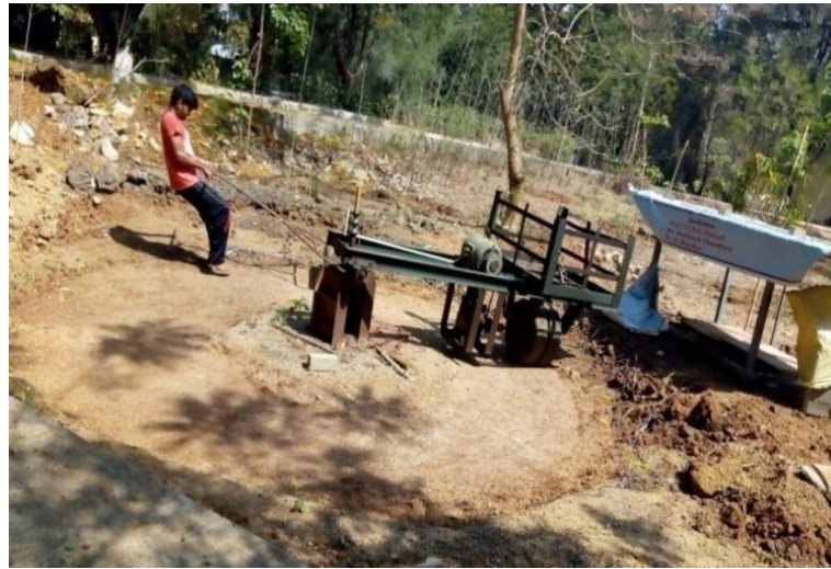
Figure 3.19 Compaction of sub-base material using the roller
