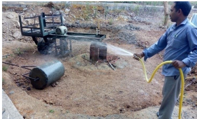
Figure 3.18 Sprinkling of water over sub-base
