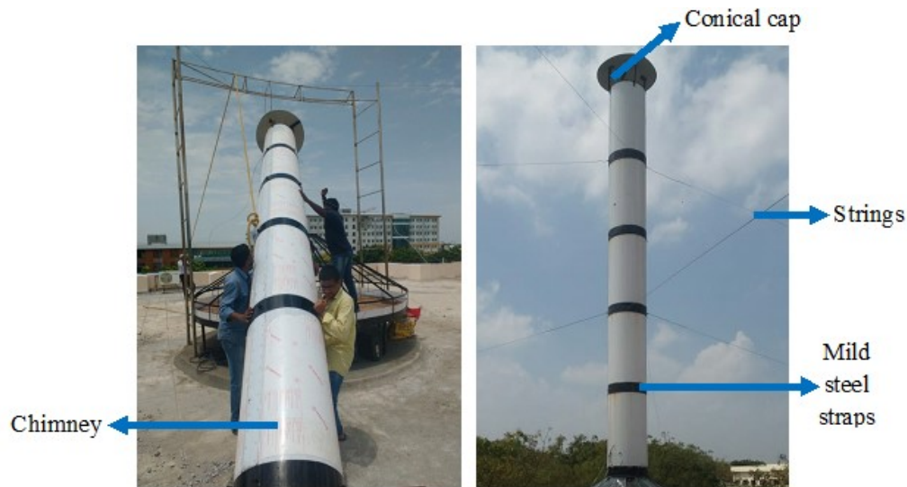
Fig. 2.16. Solar chimney (or) tower and strings
