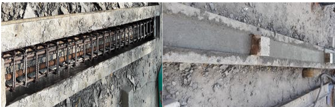
4.8 (a) Steel moulds for casting of RC beam
