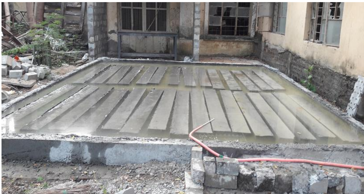
Figure 4.10 Curing of RC and FGRC beams
