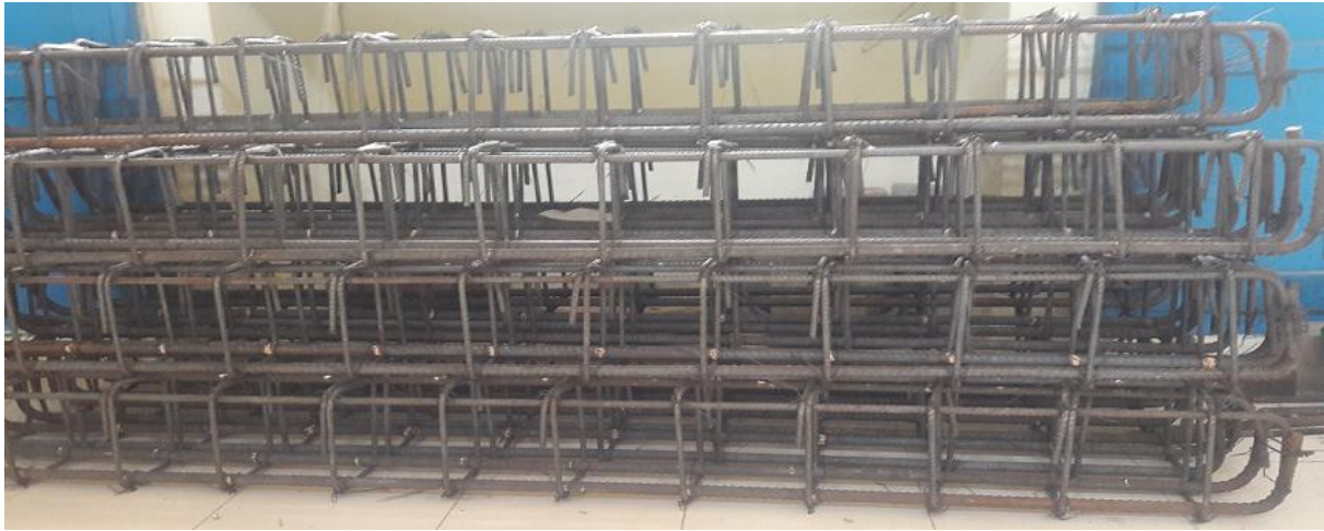
Figure 4.7 Reinforcement cages prepared for casting
