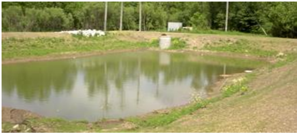
Figure 1.2 Sedimentation ponds (source: https://city.milwaukee.gov/SWMP/Erosion-Control/Advanced-Control-Measures/Sediment-Basin )
