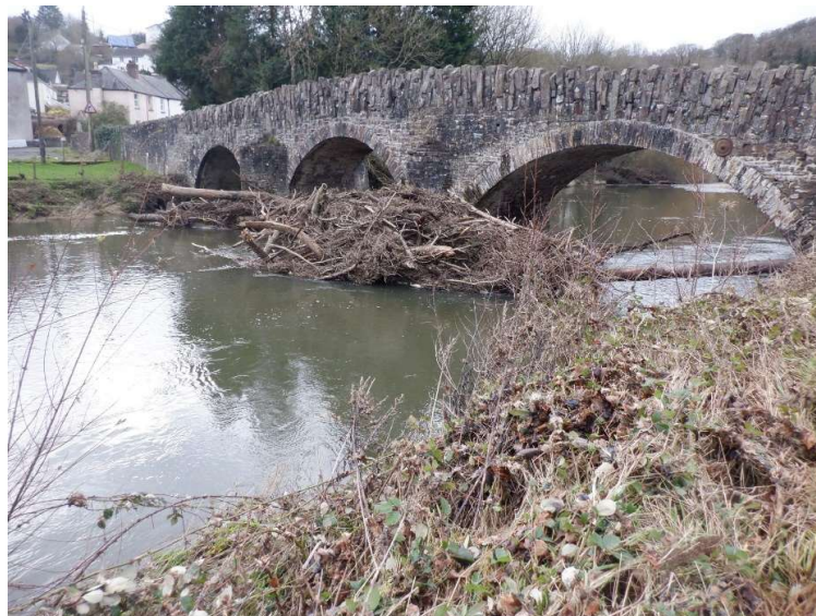
Figure 2.2 Accumulation of debris around bridge piers (Source: Jenny Knight )
