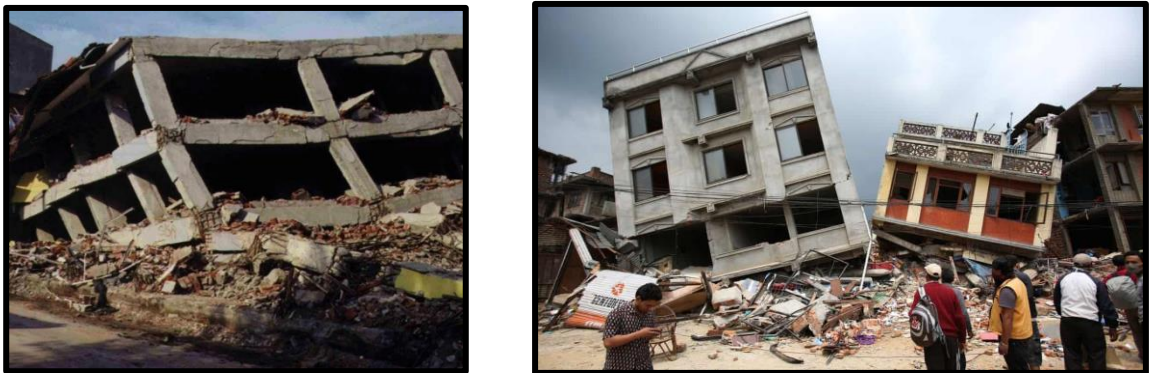
Fig. 1.1 Structural damage caused by earthquakes (Sources: Saatcioglu, 2013. Encyclopedia of Natural Hazards ; Springer; https://www.theguardian.com/cities/2015/apr/30/nepal-earthquake-disaster-building-collapse-resilience-kathmandu )
