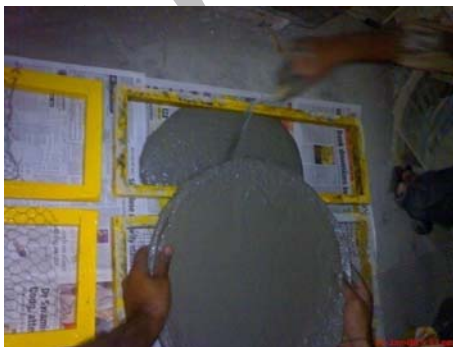
Figure 3(a). Placing of mortar into moulds
