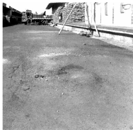
Figure 2. Shear failure of flexible pavements noticed along wheel tracks at case study area 1.
