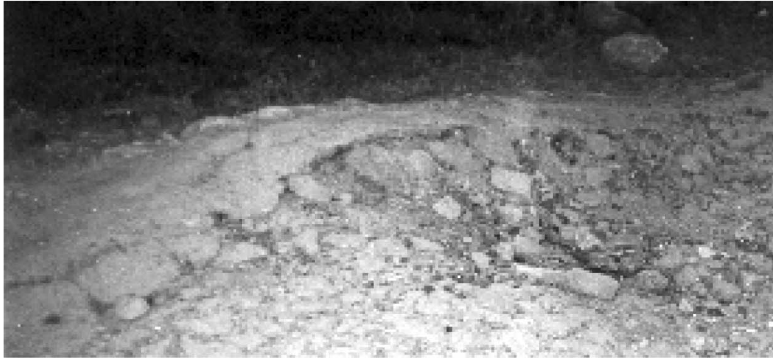
Figure 3. Shear failure of subgrade in edge region of flexible pavement at case study area 2.
